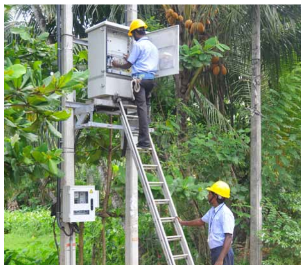
MSAN installation under the i-Sri Lanka programme
