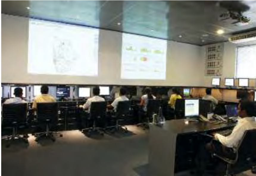
Mobitel's Integrated Network Operating Centre
